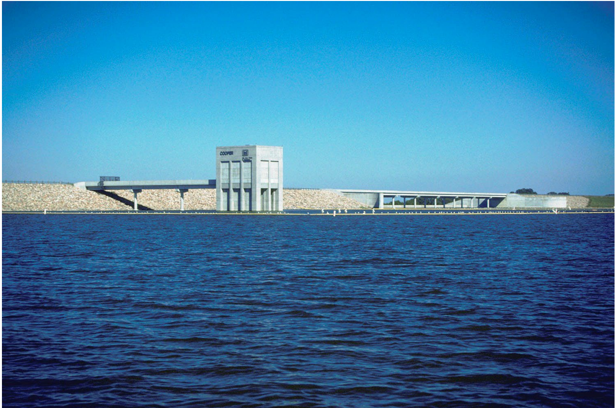
Photo 1.1 Cooper Dam at Jim Chapman Lake (USACE Photo)
