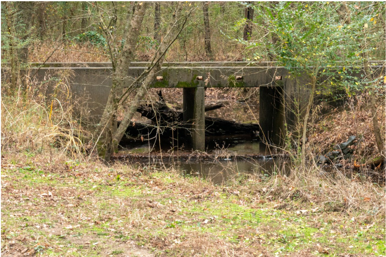
Photo 5.14 Woodland Bridge at White Oak Creek Mitigation Area (USACE photo)
