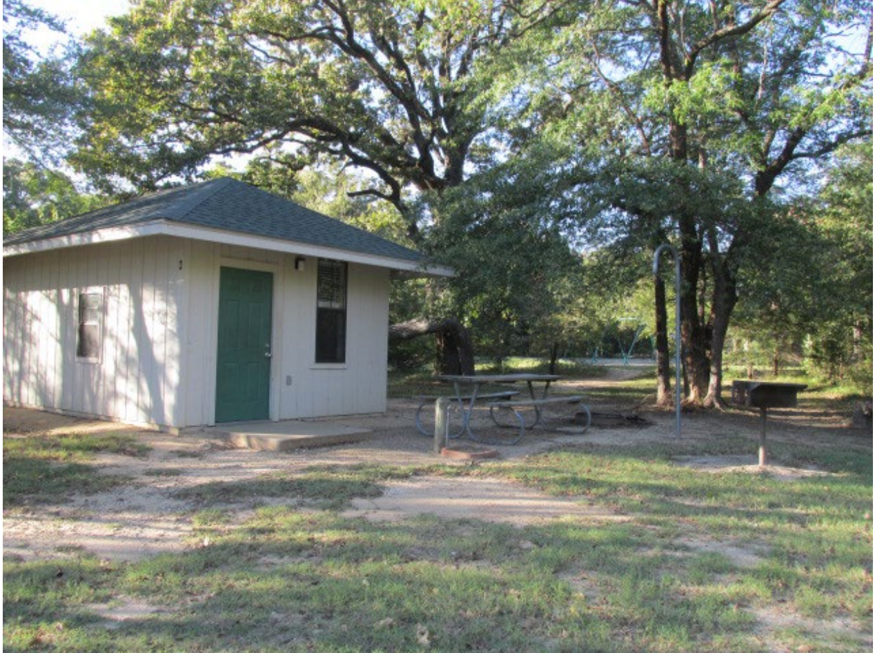
Photo 5.9 Granny's Neck shelter Area Cabin (Source: TPWD)
